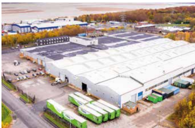
Abbey's new warehousing space offers an outlet to store goods both on a short or long-term basis
